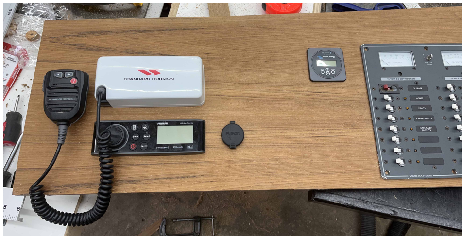
Laminating the plywood and mounting the equipment
