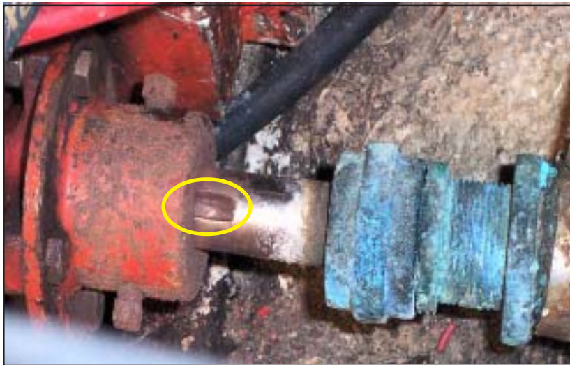
Figure 1 - Shaft coupling missing key
