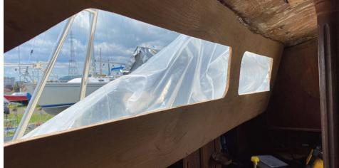
clamps was used to hold the teak to the cabin side, which was easier in the spots around the openings. We were also able to use some screws along the bottom as those would be covered by the handrails.
